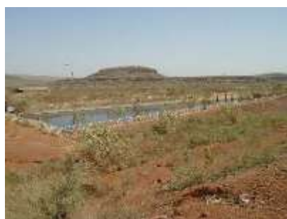
View of the cell's retention basin
